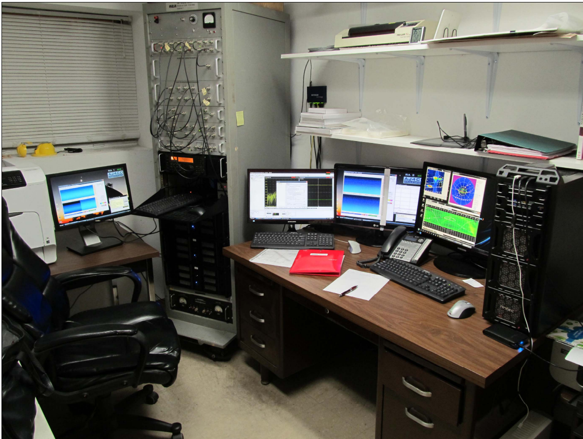
TWB installed in a 19" rack. AJ4CO Observatory, High Springs, Florida.
